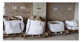
Figure 5. The construction waste is separated and collected on each floor of the construction site.
