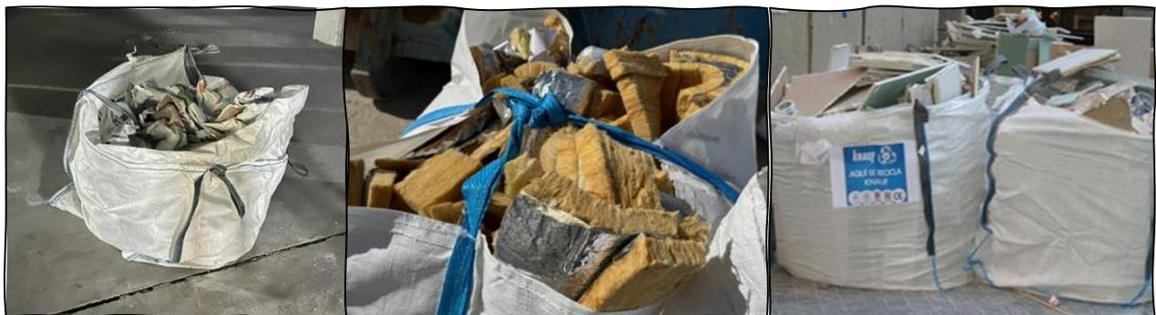
2 The next step involves the collection of the bulk bags by the **construction and demolition (C&D) waste collector**, who transports them to a designated waste management facility. This approach avoids the typical mixed waste containers which often end up in landfills, along with their associated fees.
