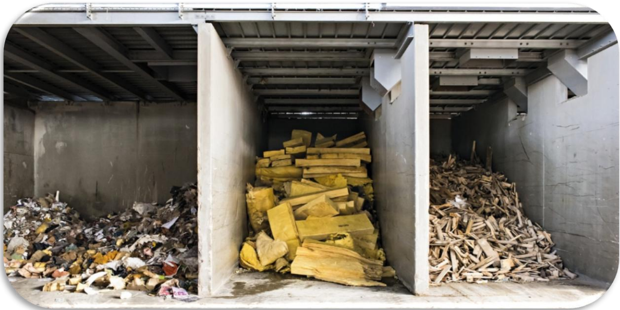
Figure 1: Segregation of materials for reuse and recycling. Saint-Gobain
